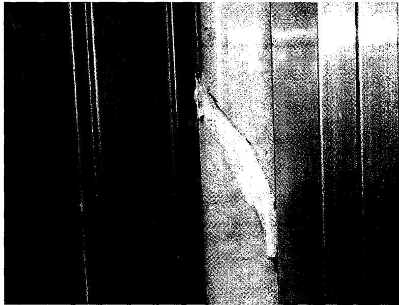
Cracks in Marble Tile
