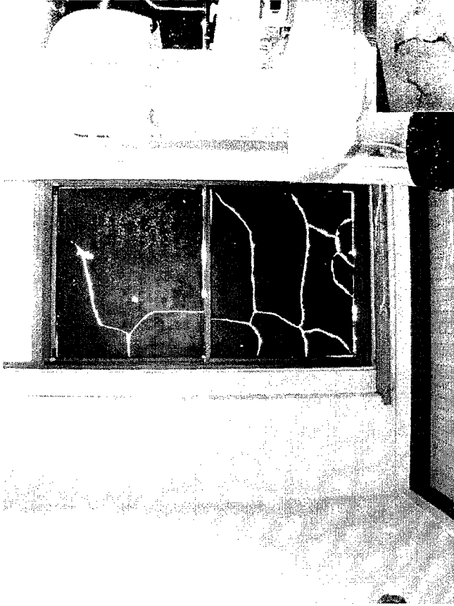
4 th floor jury men's restroom - window is painted
